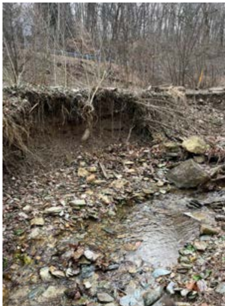
The small creek running through Jenkins' property is overwhelmed with surging runoff during storms, resulting in damaging floods and erosion, as displayed in these photos.
